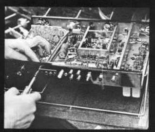
This finished unit is a rigid duplicate of a precision laboratory model. Each girl follows a precision sample when she wires. Each wire, resistor, and capacitor is wired into its specific place. Care and precision are built into each McIntosh. Each girl is responsible for her wiring area, She knows you will not settle for second best. She knows you are as demanding a customer as she is when she shops.
